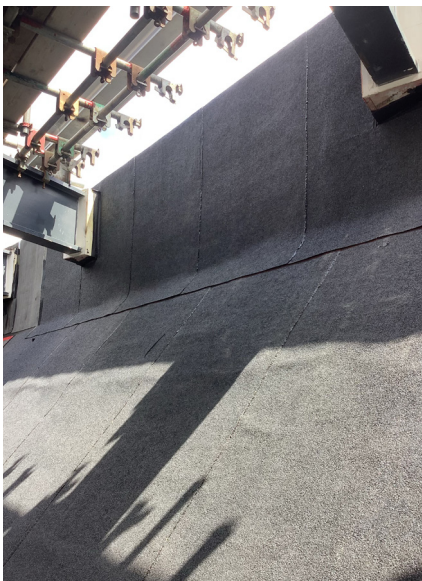
The underground plenums.
