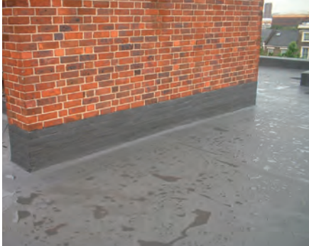
Above: Dark grey roof refurbishment
