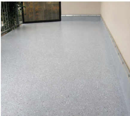
Below: New light grey balconies
