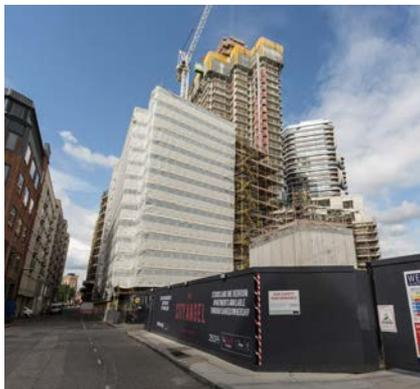
Principal Tower has been designed to reduce energy use, the tower targets the Code for Sustainable Homes Level 4, with environmental strategies including a combined heat and power plant, roof mounted photovoltaic panels and grey water harvesting, this is due for completion in 2019.
