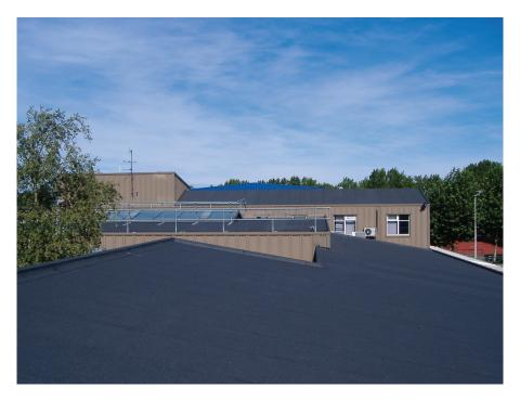
Achieving the complex refurbishment programme within the required time period required the use of a variety of **Esha Upgrade Waterproofing Systems** including self-adhesive EshaFlex 370 SA Black mineral reinforced bitumen membrane, torch applied EshaFlex 370 Black mineral reinforced bitumen membrane and cold bonded EshaUniversal single layer POCB membrane – providing the perfect solution at Kelmscott School.
