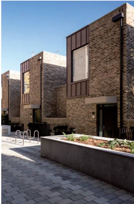
St Pancras Place (above) and Anchorage House, London (below right) both use Radmat Blue Roof systems finished with either green roofs or paving and planters.
