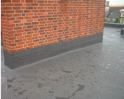
Above: Dark grey roof refurbishment
