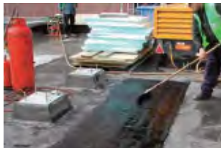
Apply 1st layer in 1m wide bays.
