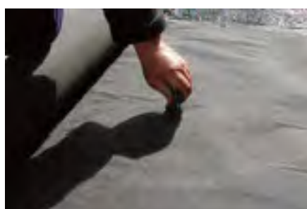
Check thickness of system.
