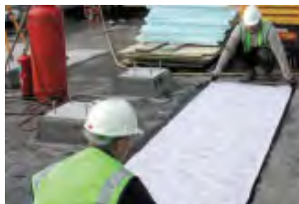
Install reinforcement layer.
