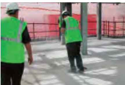
Sweep to remove debris
