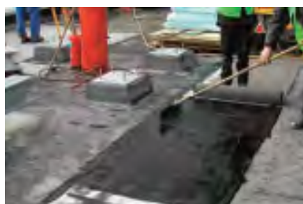
Install final layer with protection sheet.
