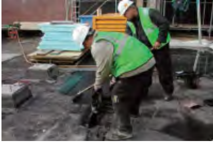
Install first layer
