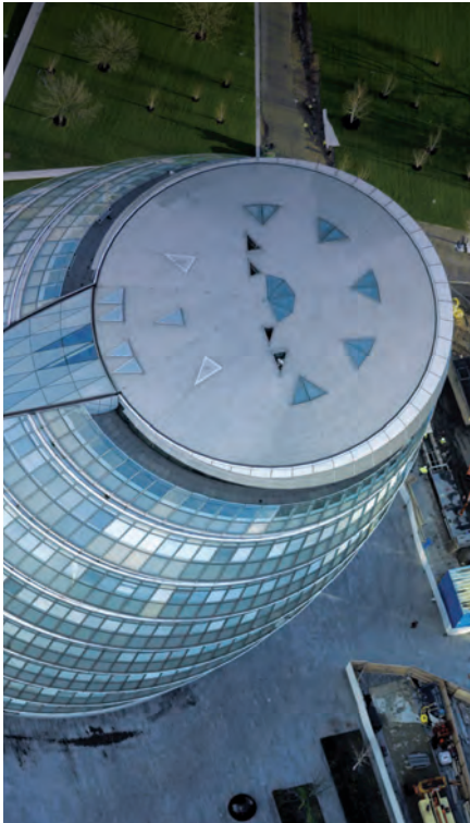
Used extensively on and around the higher terrace and over the many podium levels, PermaQuik was the waterproofing choice for City Hall, London .
