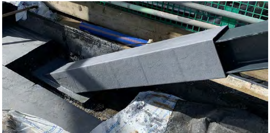
Above: ReadySeal can be applied to steel supports and pipework as part of the waterproofing system
