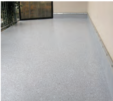
Below: New light grey balconies
