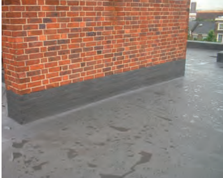
Above: Dark grey roof refurbishment
