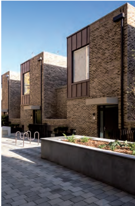
St Pancras Place (above) and Anchorage House, London (below right) both use Radmat Blue Roof systems finished with either green roofs or paving and planters.
