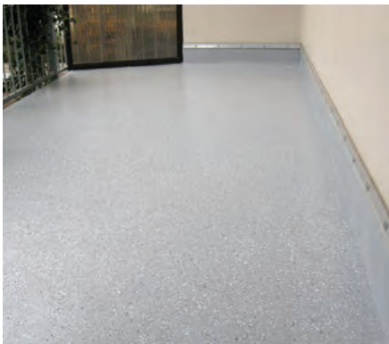
Below: New light grey balconies
