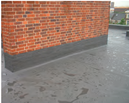
Above: Dark grey roof refurbishment
