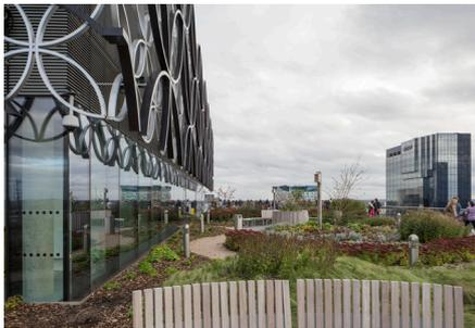
Radmat Approved Contractor Prater delivered a roofing solution that is BBA Certified to last 'the life of the building'. Consisting of Radmat **PermaQuik PQ6100** Hot Melt Monolithic waterproofing membrane, **Root Resistant Cap Sheet** and **ProTherm** inverted roof insulation, the entire roof was electronically tested for integrity prior to the installation of aluminum powder coated cappings to the perimeter roof upstands.
