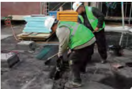
Install first layer
