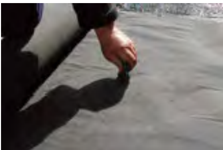
Check thickness of system.
