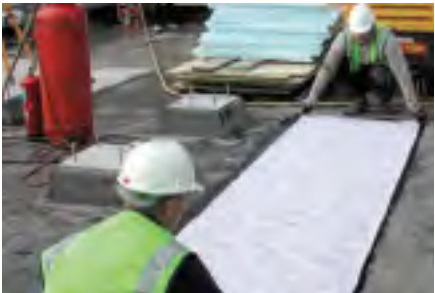
Install reinforcement layer.
