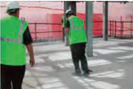
Sweep to remove debris
