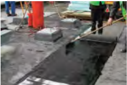
Install final layer with protection sheet.
